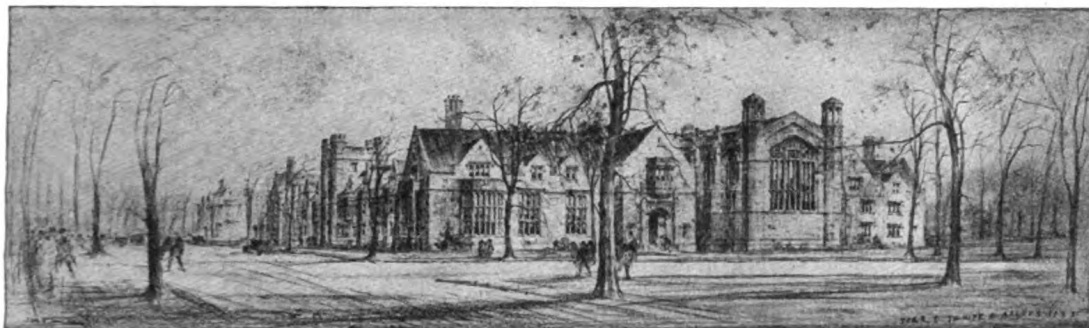
A CLOSER VIEW OF THE LAWYERS' CLUB Showing the State Street Side, and the Large Hall or Commons. York and Sawyer, Architects.
