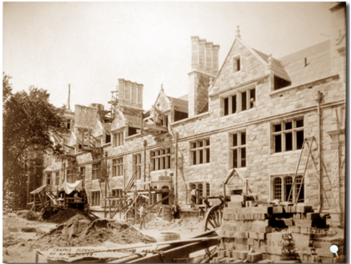
Lawyers Club under construction
