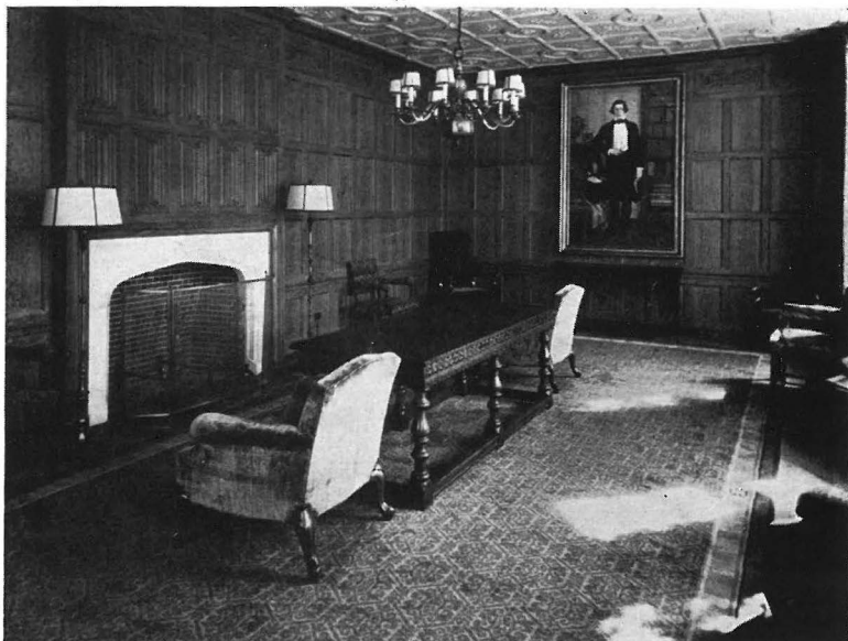
John Poller Cook Memorial Room in John P. Cook dormitory.
