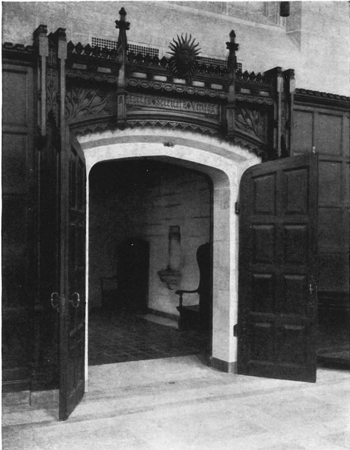
Doorway in dining room—to the lobby.
